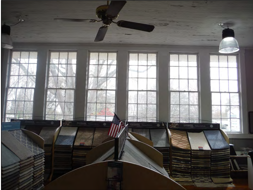
Figure 2.5.11. Interior view of Caldwell Rosenwald School, window detail, south.
