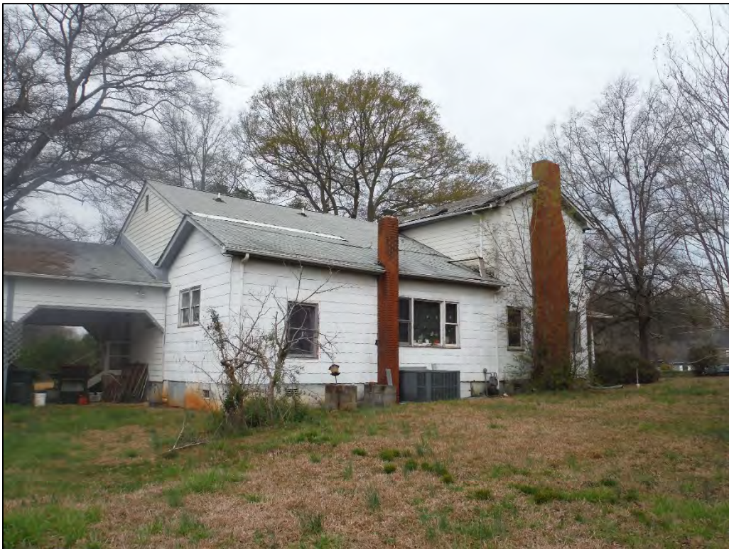
Figure 2.7.6. Houser House, residence, facing northwest.
