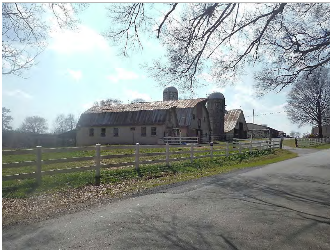
Figure 2.10.19. Stillwell-Hubbard Farm Buildings, facing southwest.
