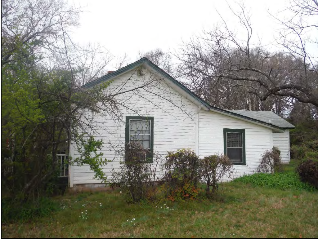
Figure 2.9.4. Brown House, facing northwest.
