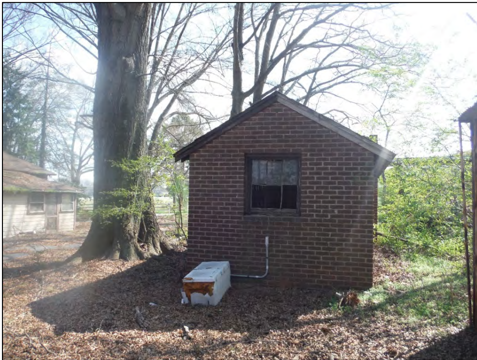
Figure 2.10.10. Stillwell-Hubbard House, storage building, facing south.
