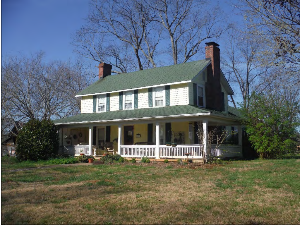
Figure 2.1.24. House at 1287 Rufus Road, facing southwest.
