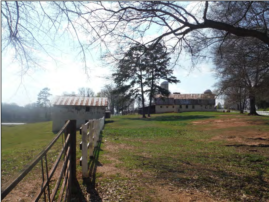
Figure 2.10.28. Stillwell-Hubbard Farm Buildings, facing west.
