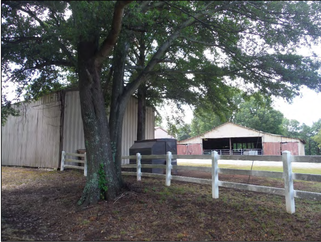
Figure 2.10.24. Stillwell-Hubbard Farm Buildings, facing south.
