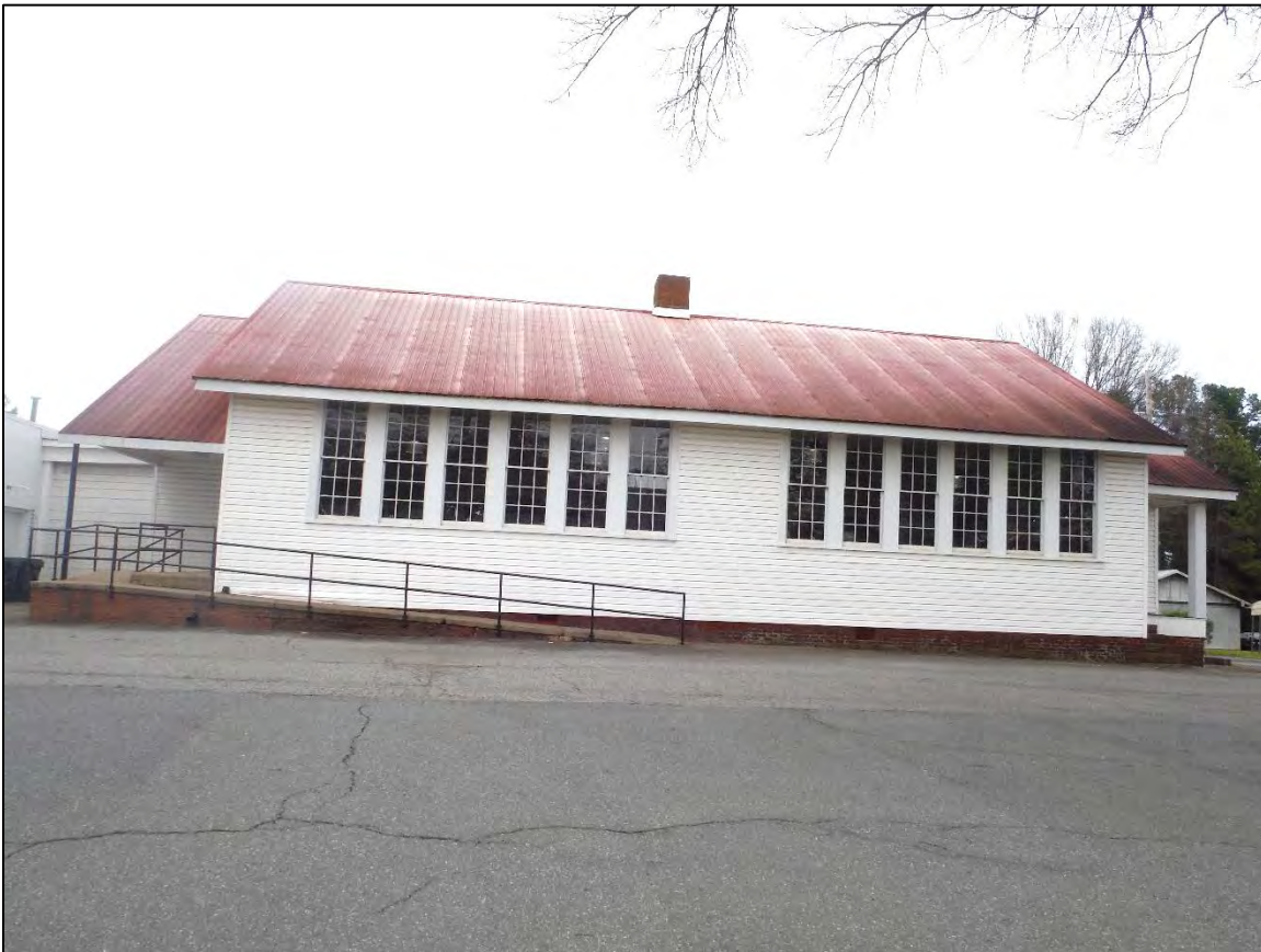
Figure 2.5.1. View of Caldwell Rosenwald School, facing northwest.
