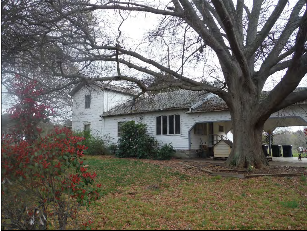
Figure 2.7.5. Houser House, residence, facing northeast.
