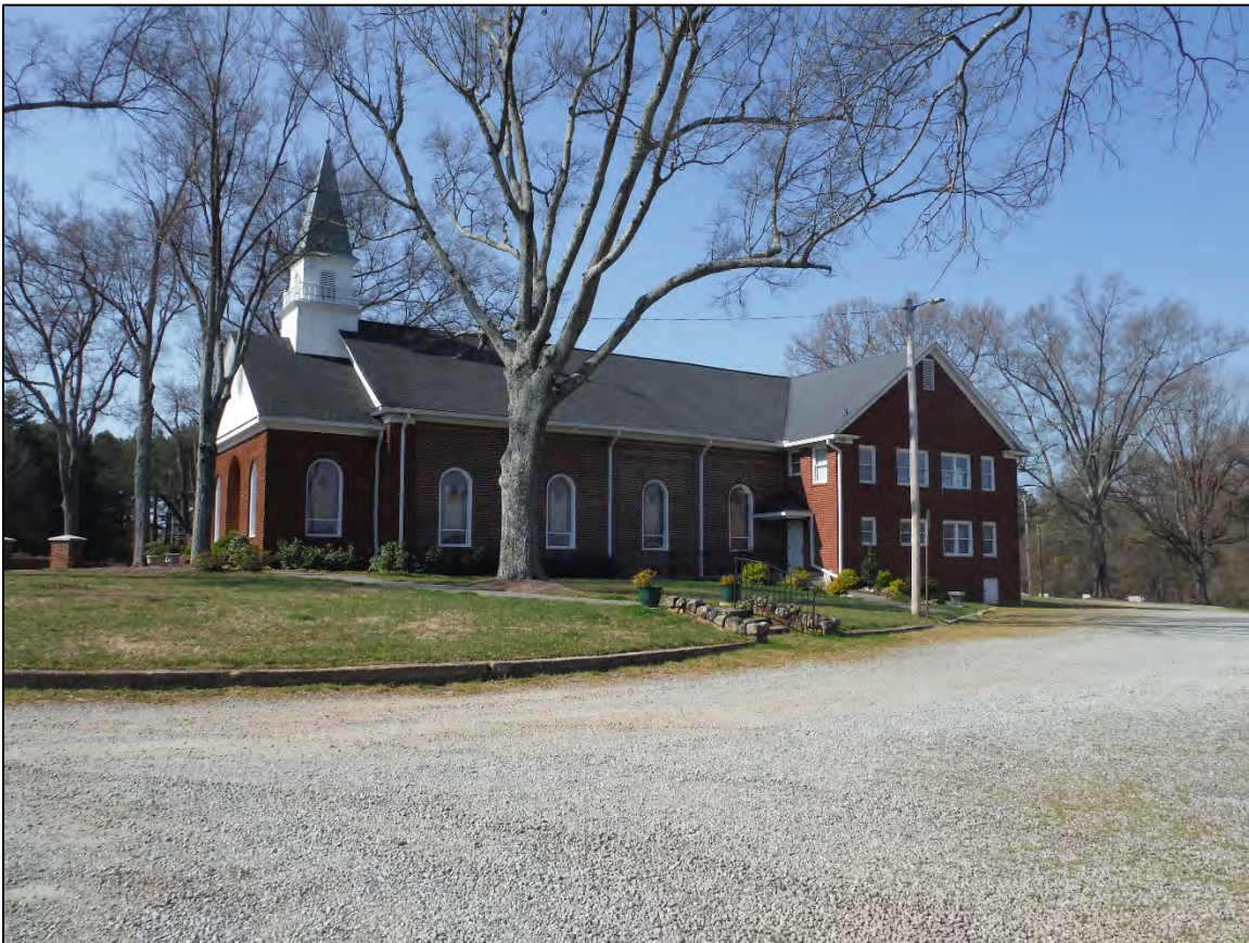
Figure 2.6.1. View of Gilead ARP Church, facing southwest.
