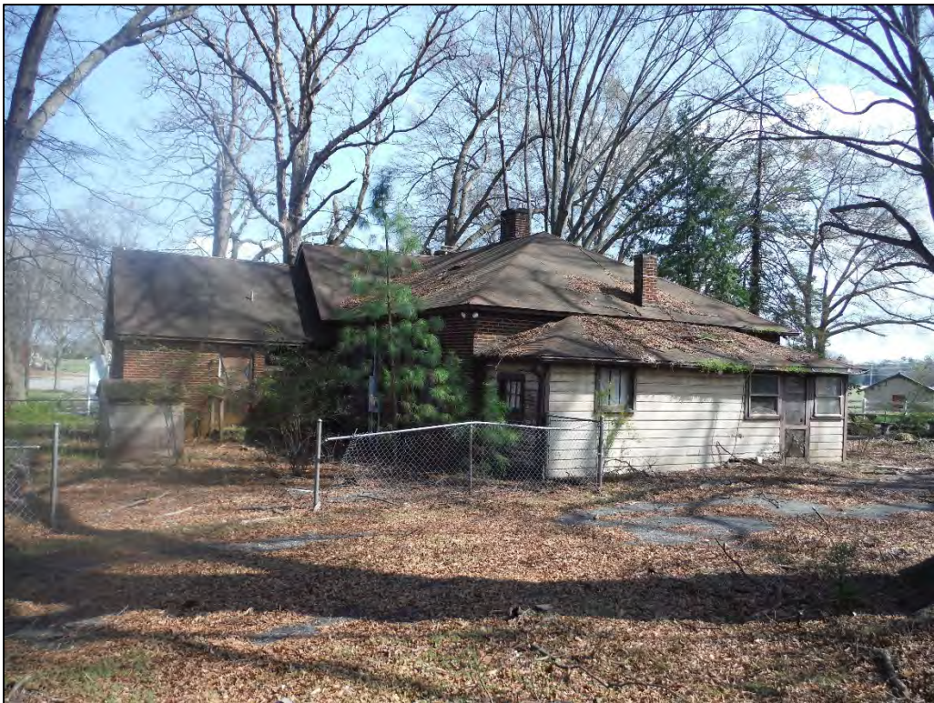
Figure 2.10.6. Stillwell-Hubbard House, facing southeast.
