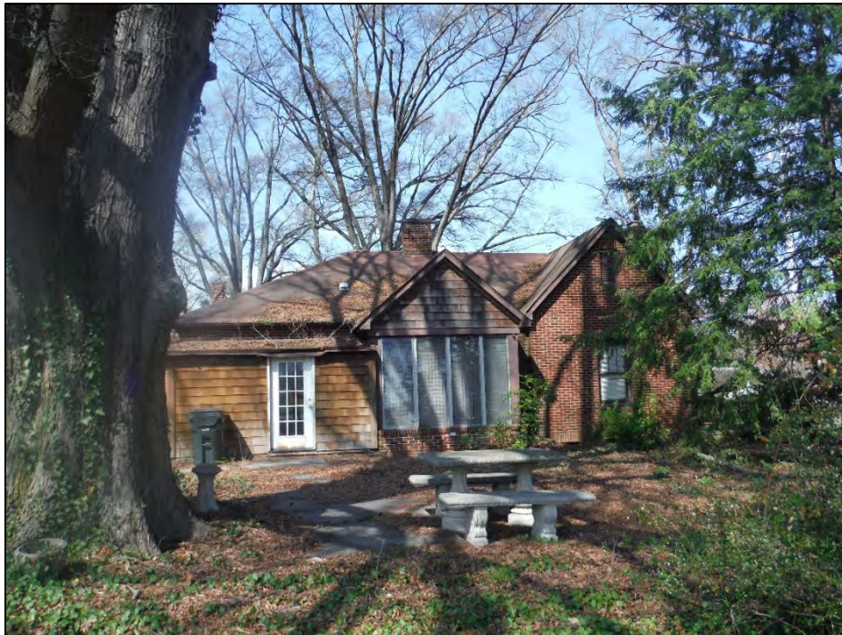
Figure 2.10.4. Stillwell-Hubbard House, facing northeast.
