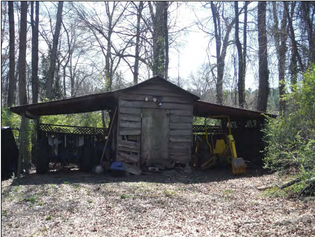
Figure 2.3.16. View of equipment storage building, Lynn Beard House, facing southwest.
