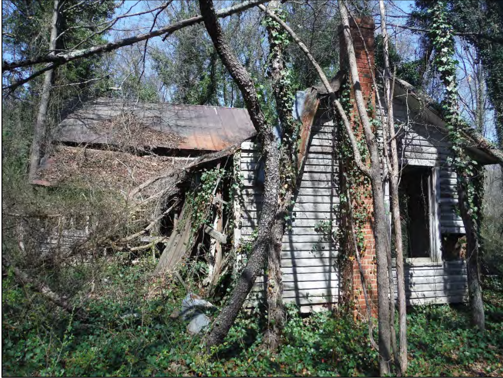
Figure 2.2.5. View of the Carl Beard House, facing north.
