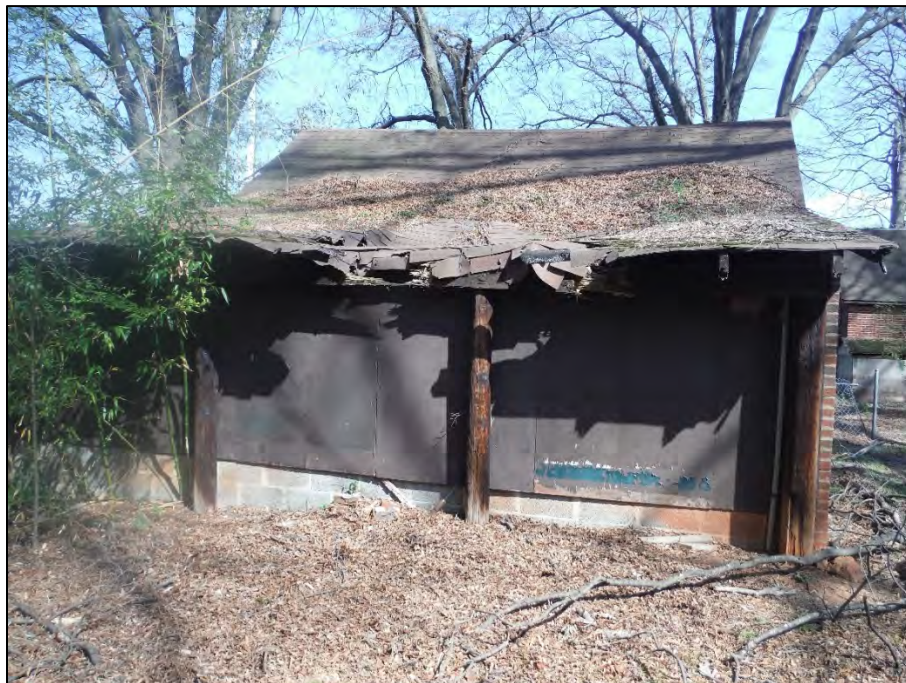
Figure 2.10.8. Stillwell-Hubbard House, garage, facing east.
