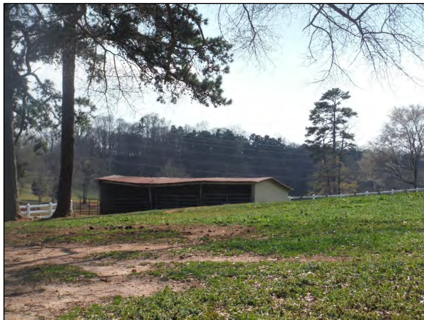
Figure 2.10.26. Stillwell-Hubbard Farm Buildings, facing southwest.
