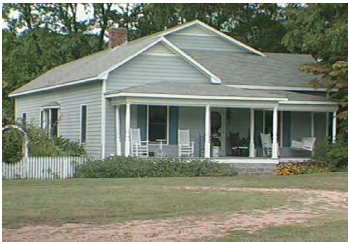
Figure 2.11.21. Historic photograph (2010) showing the Hubbard-Browning House.
