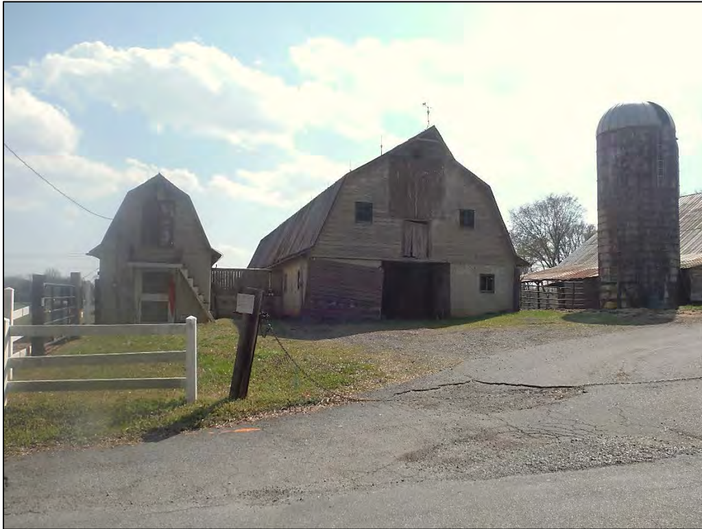
Figure 2.10.20. Stillwell-Hubbard Farm Buildings, facing south.
