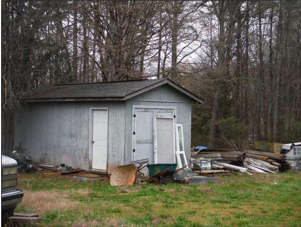
Figure 2.7.19. View of Houser House, shed, facing southwest.
