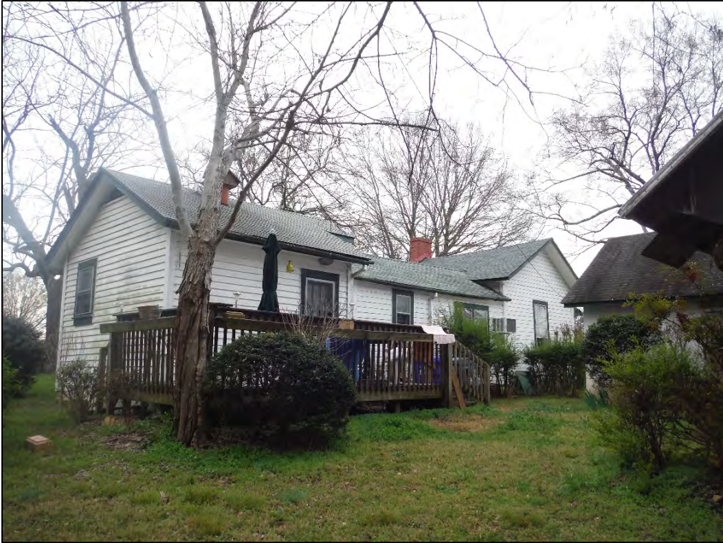
Figure 2.9.6. Brown House, facing south.
