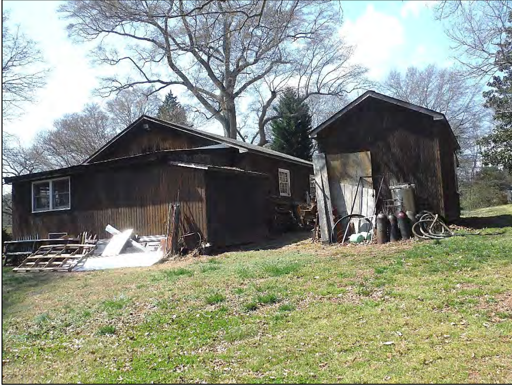
Figure 2.3.8. View of the garage and storage building, Lynn Beard House, facing northwest.
