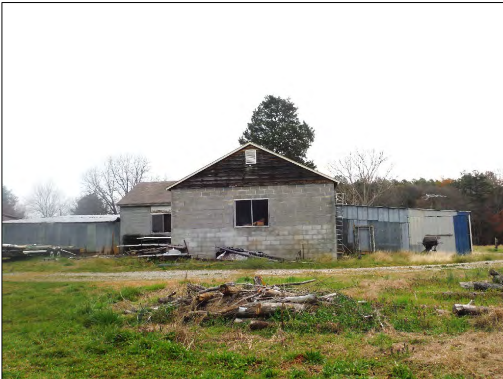
Figure 2.7.13. View of Houser House, rear of storage/workshop buildings, facing east.
