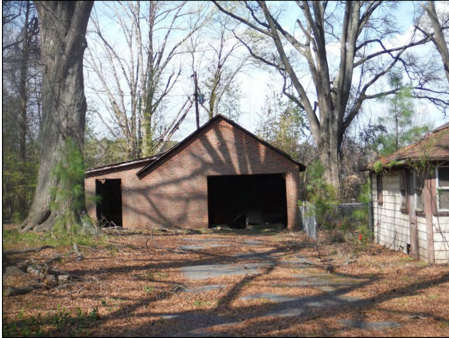
Figure 2.10.7. Stillwell-Hubbard House, garage, facing north.
