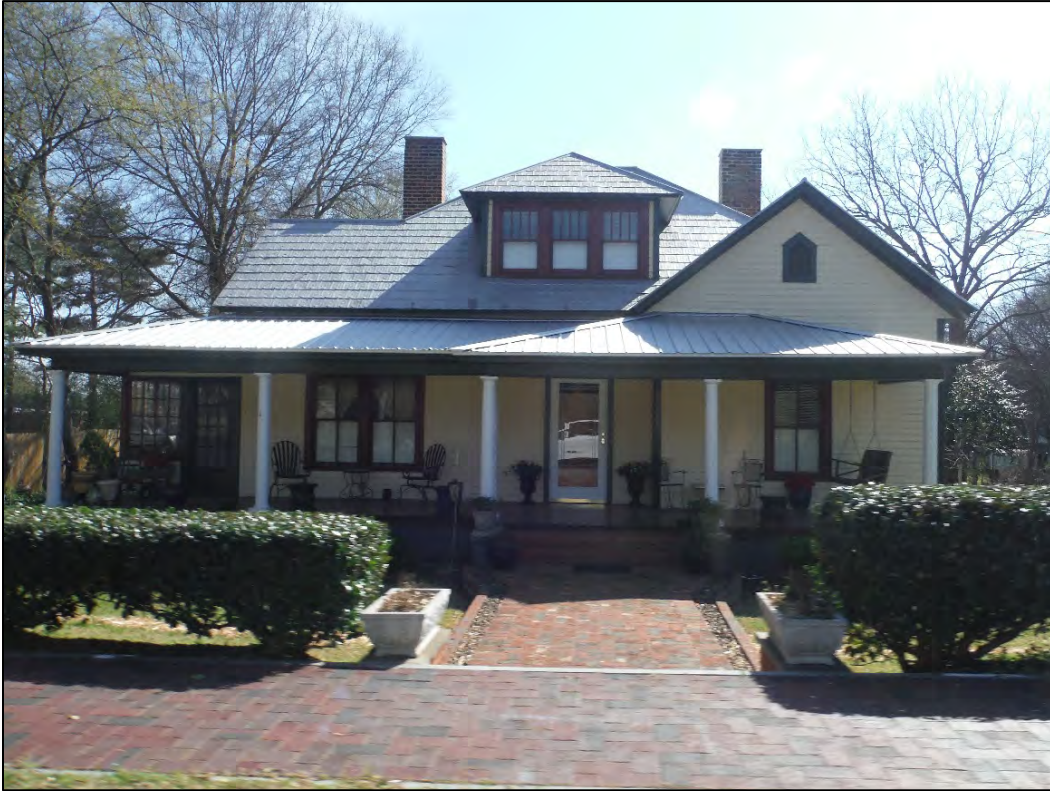
Figure 2.8.14. Howard House (MK1423), facing south.
