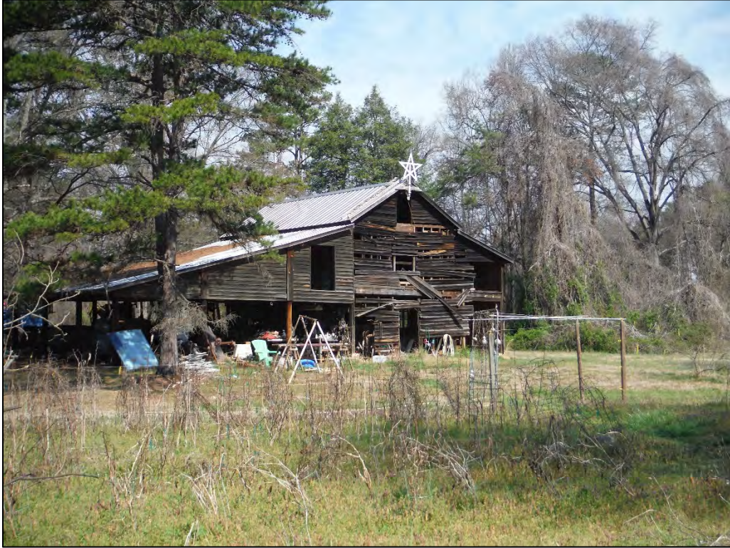
Figure 2.11.13. Hubbard-Browning House, barn, facing northeast.
