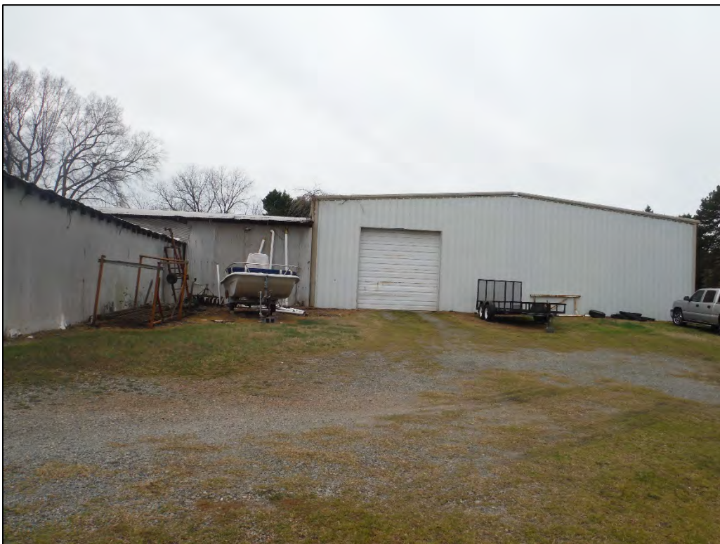
Figure 2.5.10. Caldwell Rosenwald School, rear warehouse addition, facing west.
