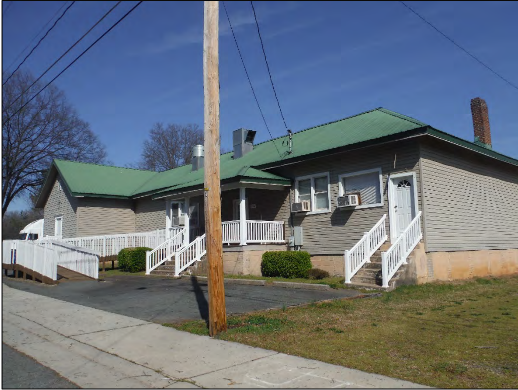
Figure 2.5.24. Smithville Rosenwald School (MK2403), facing northeast.
