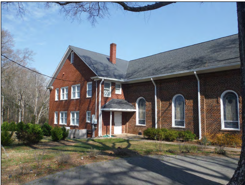
Figure 2.6.6. View of Gilead ARP Church, education wing and original structure, facing northwest.
