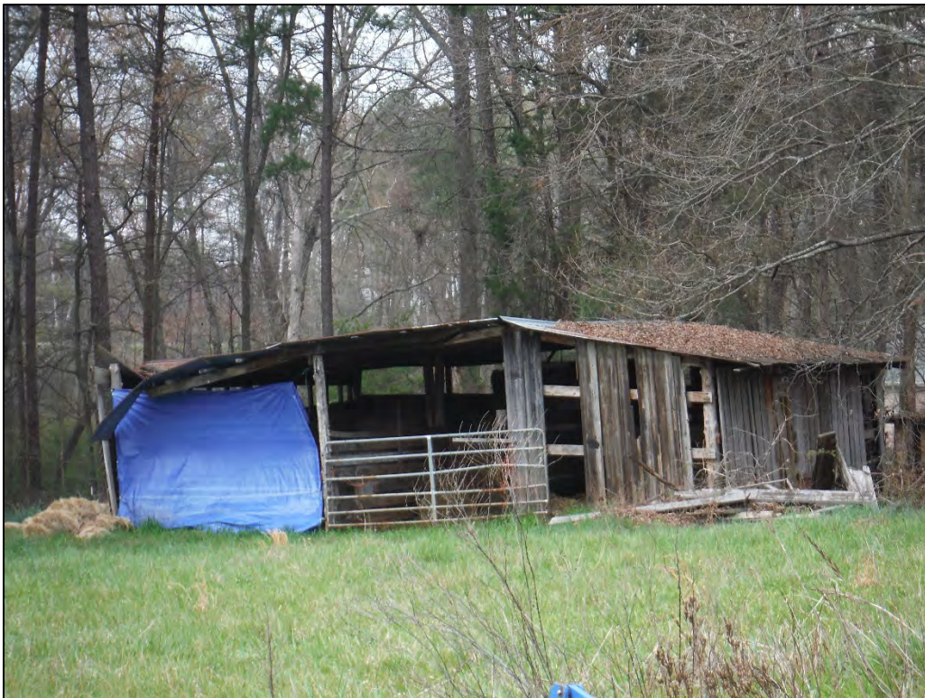
Figure 2.7.18. View of Houser House, hay storage, facing southwest.
