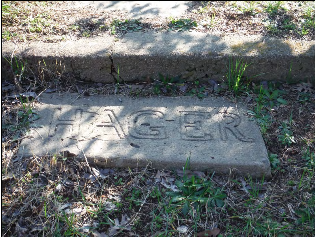
Figure 2.1.7. View of the carved stone along walkway west of J. P. Hager House, facing east.
