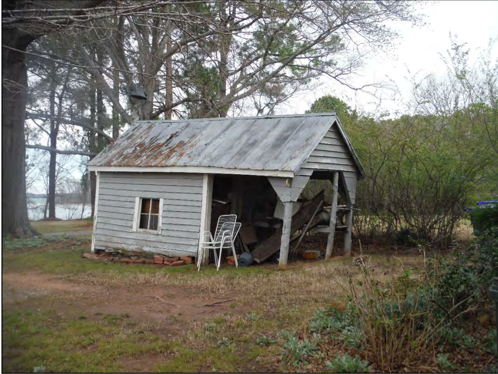
Figure 2.4.9. Blythe Homestead, well house, facing north.
