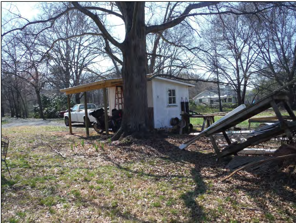
Figure 2.11.11. Hubbard-Browning House, shed, facing southeast.
