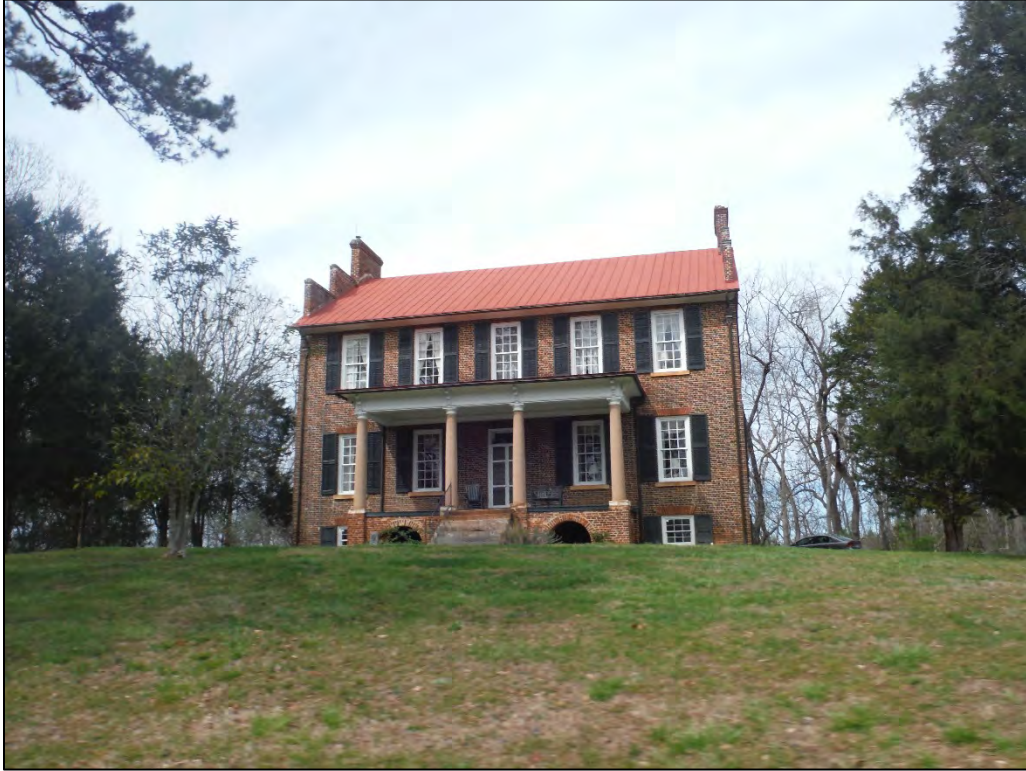
Figure 2.4.15. Cedar Grove (MK0004), facing north.
