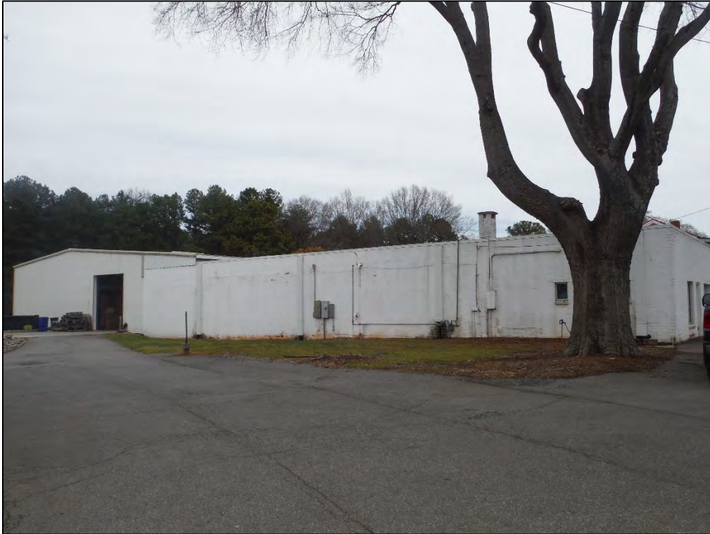
Figure 2.5.9. Caldwell Rosenwald School, side and rear warehouse additions, facing south.
