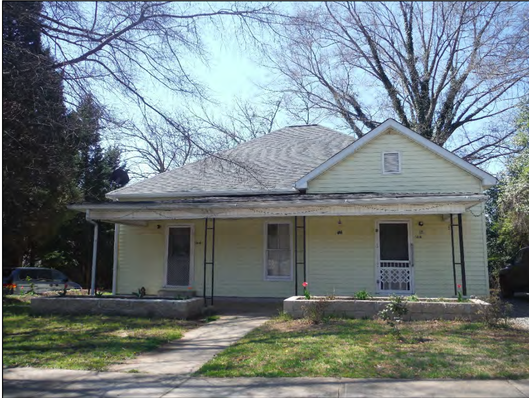
Figure 2.11.26. House at 504 South Main Street, Huntersville, (MK3568), facing south.
