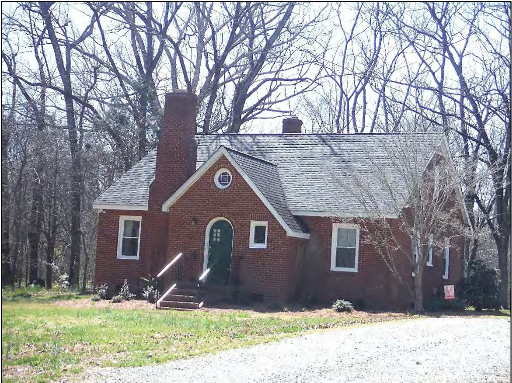
Figure 2.10.38. House at 10801 Beatties Ford Road (NSN), facing west.
