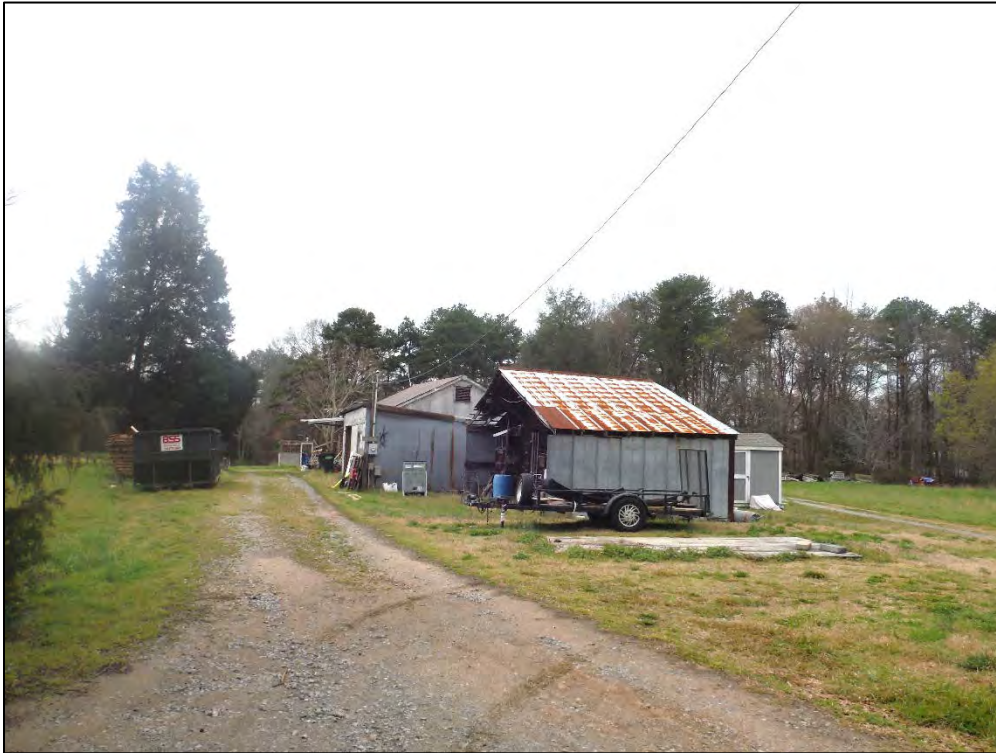
Figure 2.7.8. View of Houser House, outbuildings, facing south.
