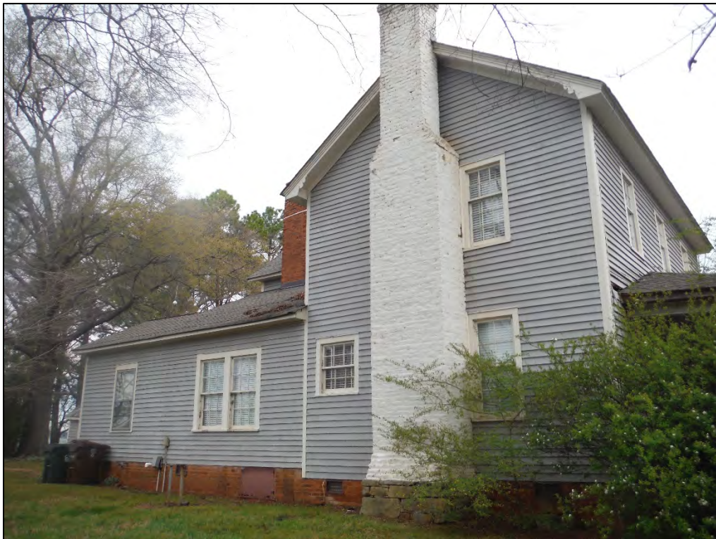
Figure 2.4.7. Blythe Homestead, residence, facing north.
