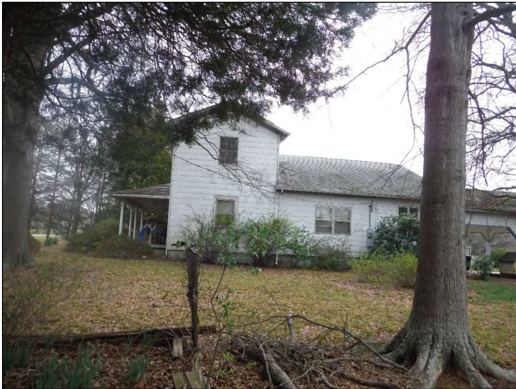
Figure 2.7.4. Houser House, residence, facing east.
