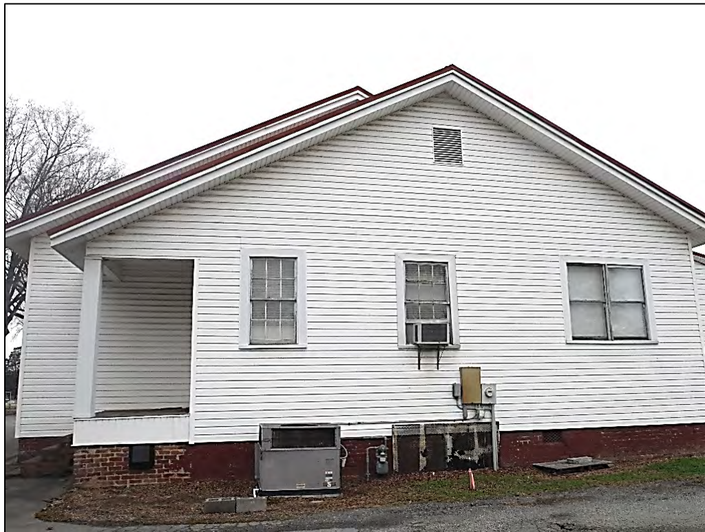
Figure 2.5.4. Caldwell Rosenwald School, facing southwest.
