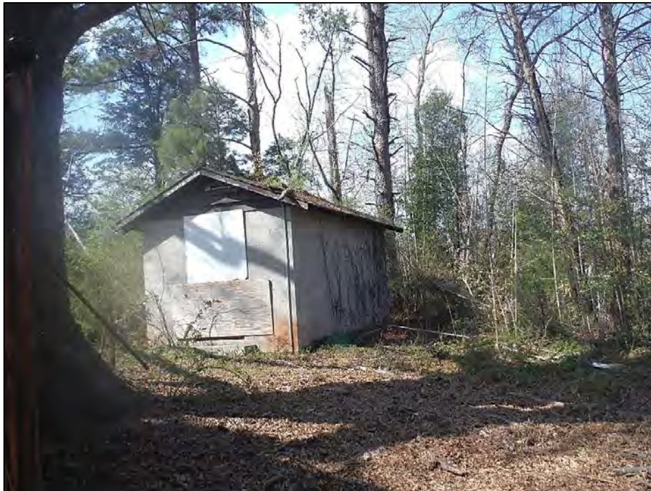
Figure 2.10.12. Stillwell-Hubbard House, storage building, facing north.
