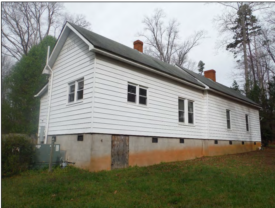
Figure 2.8.4. Long-Hastings house, facing northwest.
