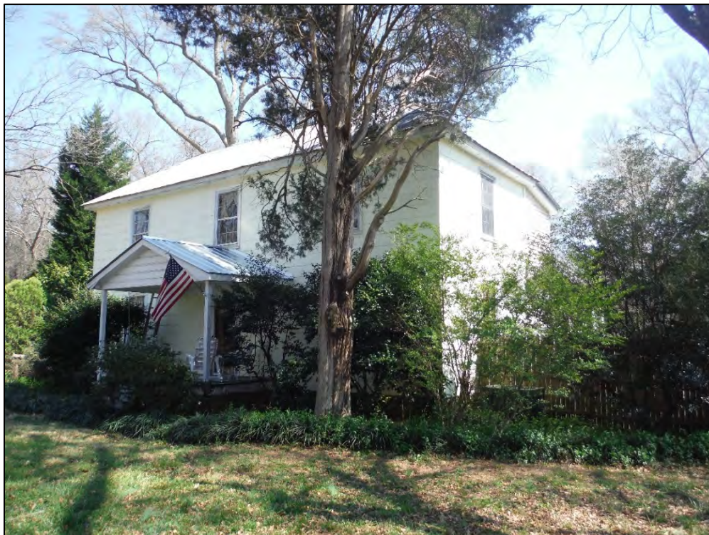
Figure 2.3.3. View of the Lynn Beard House, facing northeast.
