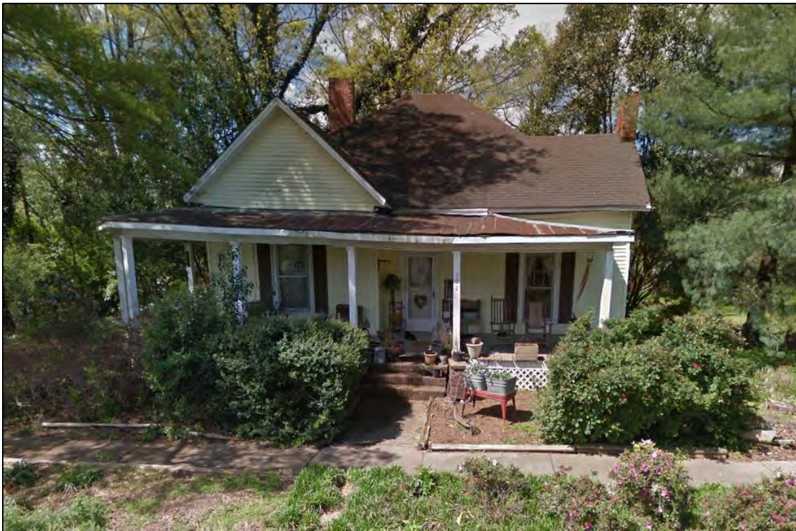
Figure 2.11.25. House at 502 South Main Street, Huntersville (MK1377), facing west.
