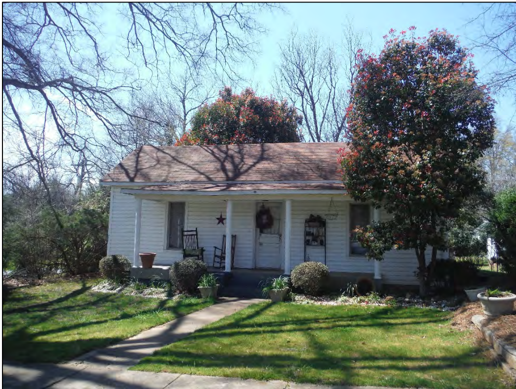
Figure 2.9.11. House at 406 South Main Street, Huntersville (MK3569), facing west.
