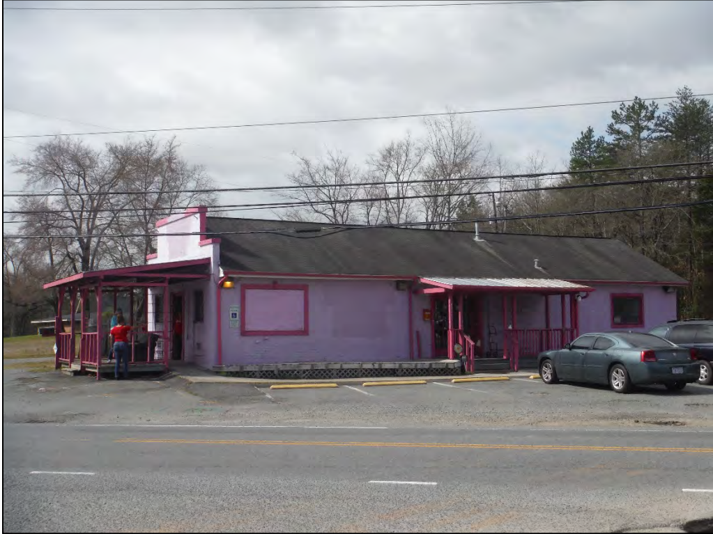
Figure 2.10.40. Store at 3601 Oakdale Road (NSN), facing southwest.
