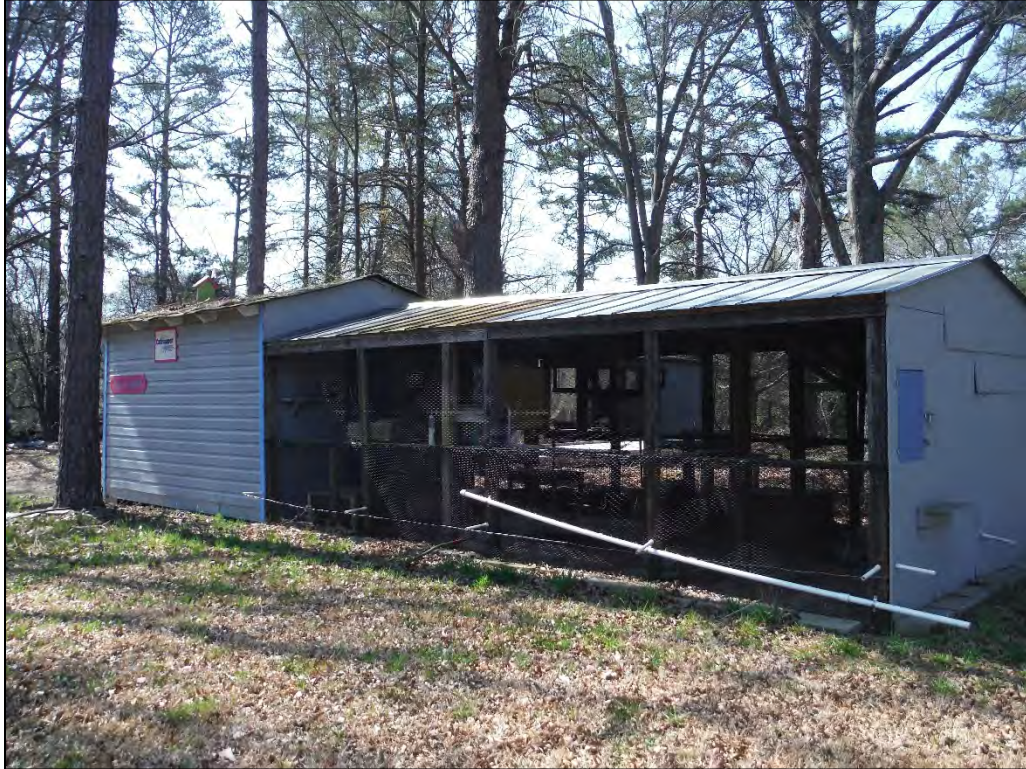
Figure 2.11.17. Hubbard-Browning House, cat house, facing south.
