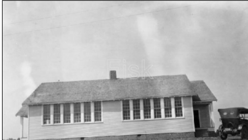
Figure 2.5.18. Historic photograph of the Caldwell Rosenwald School, south elevation (Fisk University 2001).
