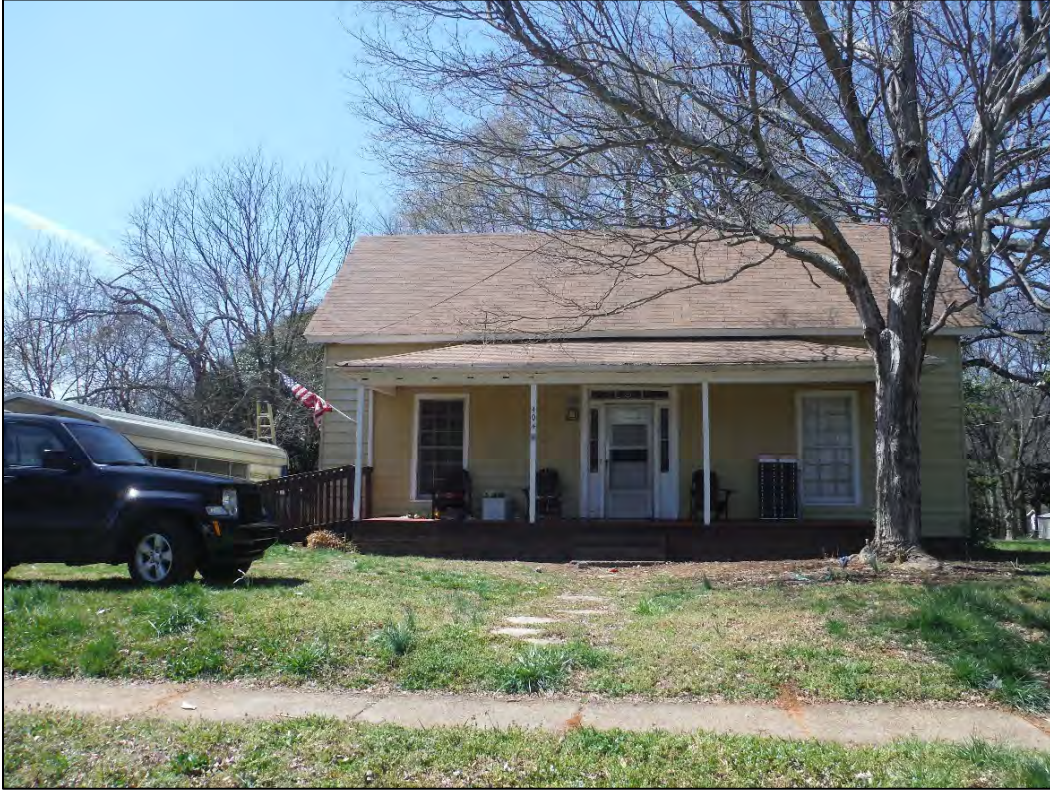
Figure 2.9.12. House at 404 South Main Street, Huntersville (MK3570), facing west.
