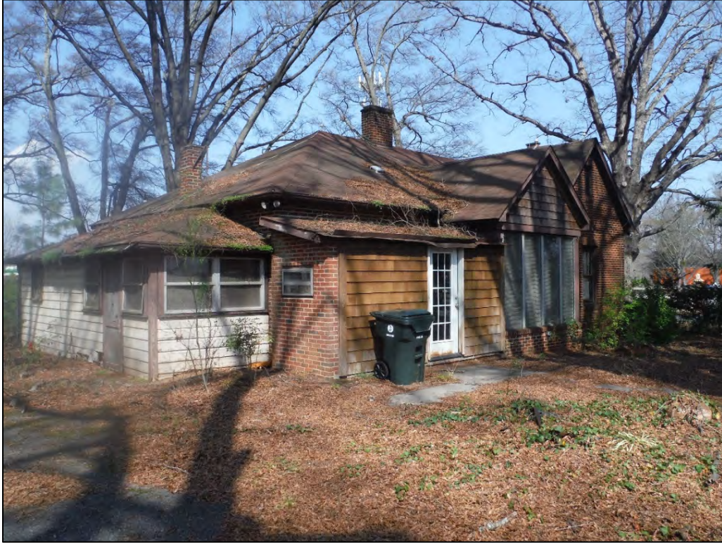
Figure 2.10.5. Stillwell-Hubbard House, facing east.
