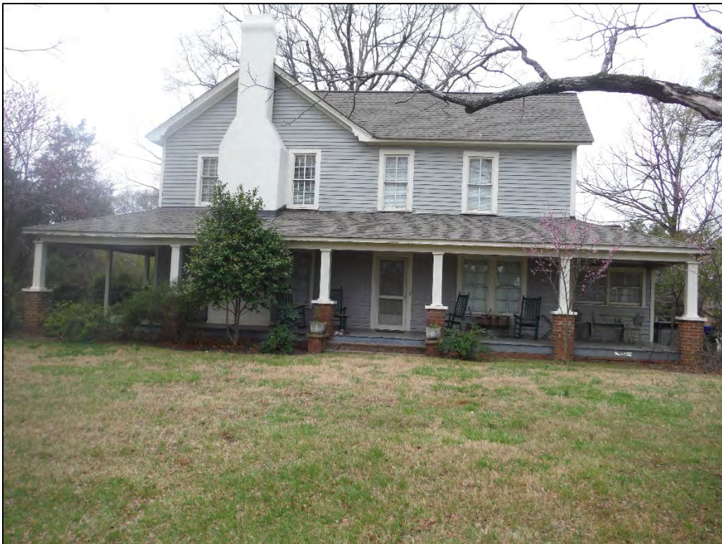
Figure 2.4.4. Blythe Homestead, residence, facing southwest.
