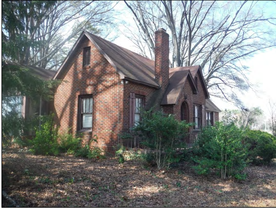
Figure 2.10.3. Stillwell-Hubbard House, facing north.
