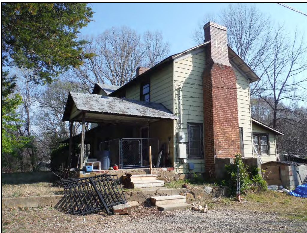
Figure 2.1.6. View of the J. P. Hager House, facing northeast.
