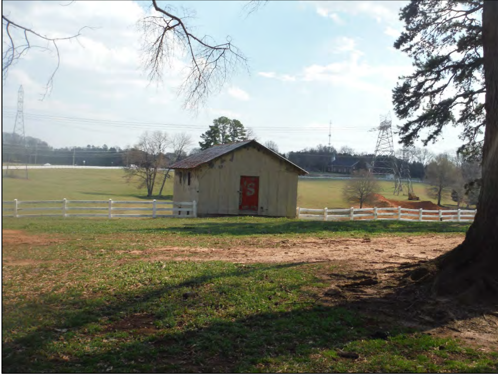
Figure 2.10.27. Stillwell-Hubbard Farm Buildings, facing south.
