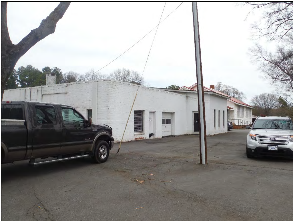
Figure 2.5.8. Caldwell Rosenwald School and side warehouse addition, facing northeast.
