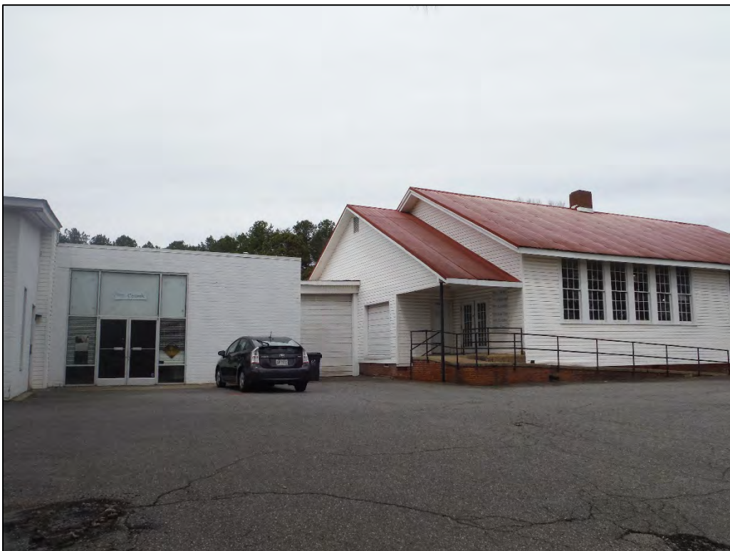
Figure 2.5.6. Caldwell Rosenwald School and side warehouse addition, facing north.
