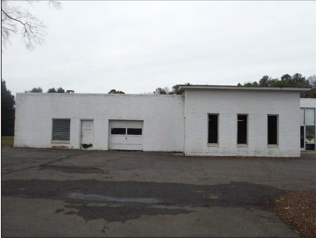
Figure 2.5.7. Caldwell Rosenwald School, side warehouse addition, facing north.
