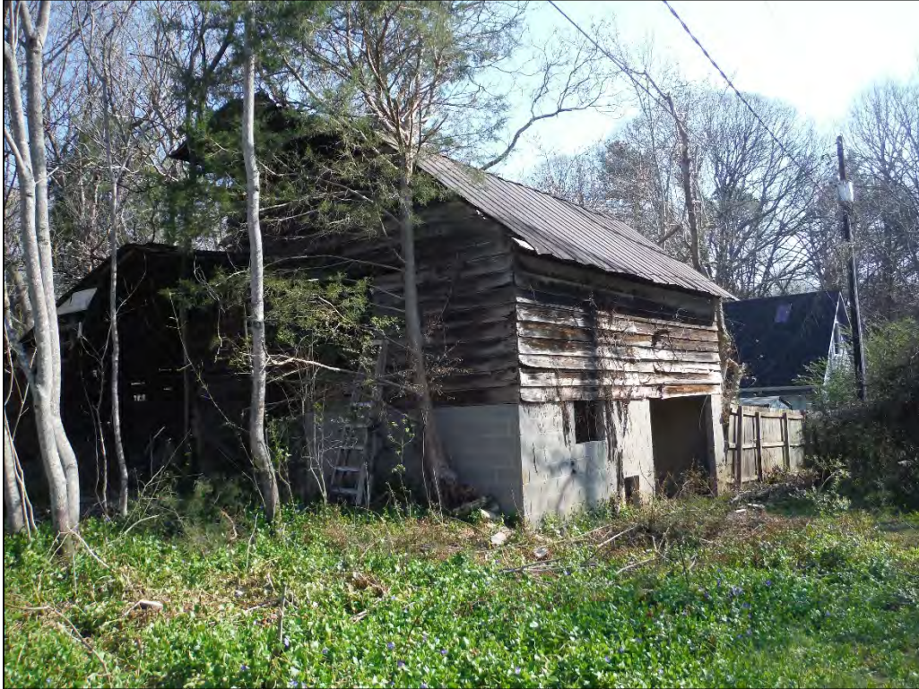
Figure 2.1.14. View of mid-twentieth-century barn, J. P. Hager House, facing northeast.
