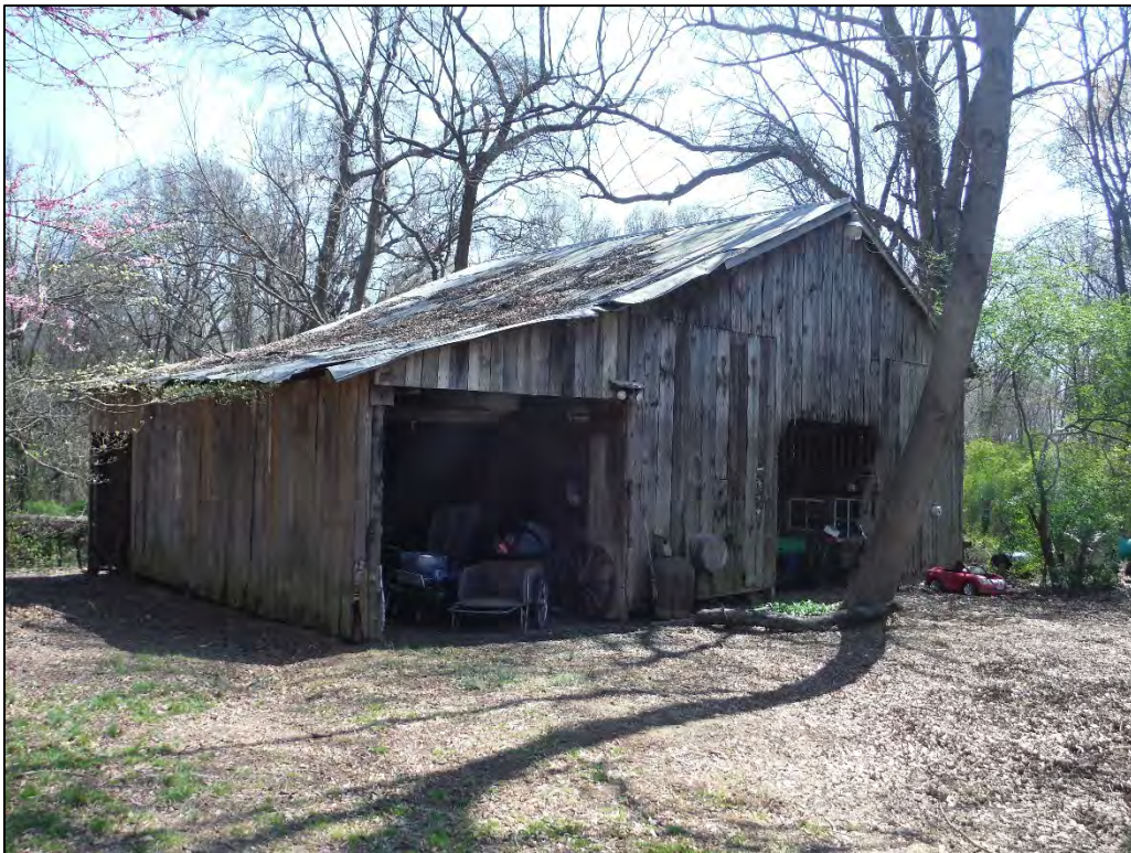
Figure 2.3.14. View of barn, Lynn Beard House, facing south.
