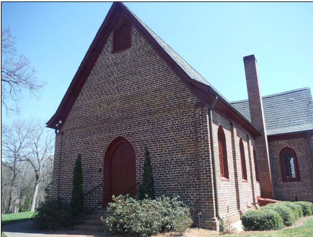
Figure 2.6.19. St. Marks Episcopal Church (MK0199), facing northeast.
