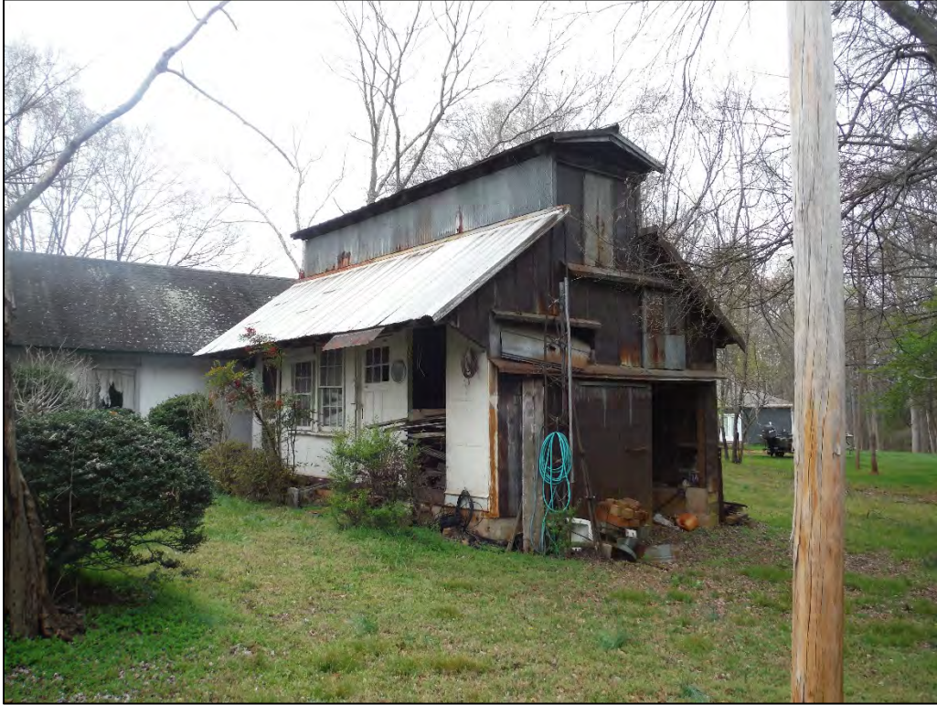
Figure 2.9.10. Brown House, bath house attached to garage, facing southwest.
