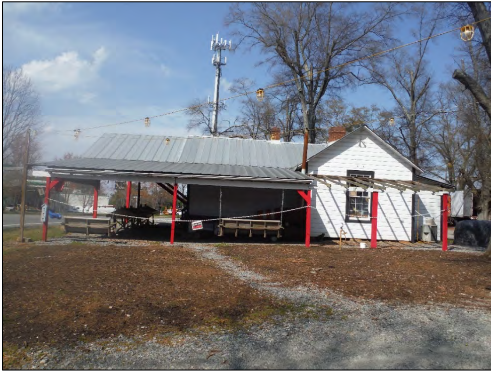
Figure 2.10.14. Stillwell-Hubbard Store, facing northeast.
