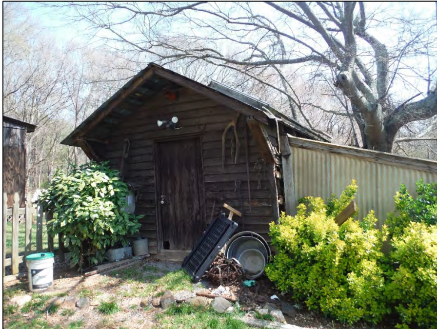
Figure 2.3.10. View of smokehouse, Lynn Beard House, facing east.
