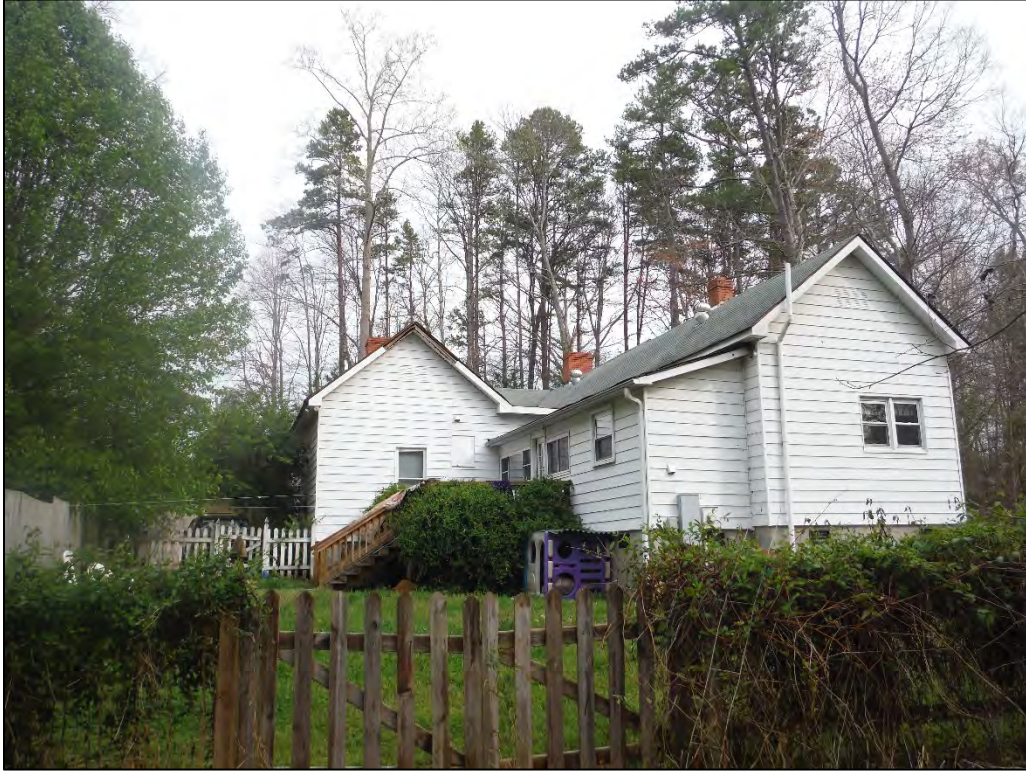
Figure 2.8.5. Long-Hastings House, facing north.
